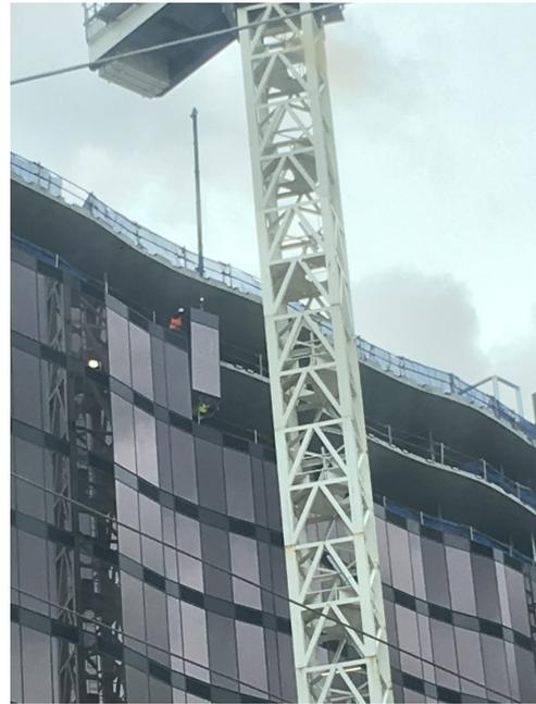
**Figure 2.2:** Conventional direct UCW installation method: Transitioning from the vertical transport task to the alignment task (photo by author, 2019).
