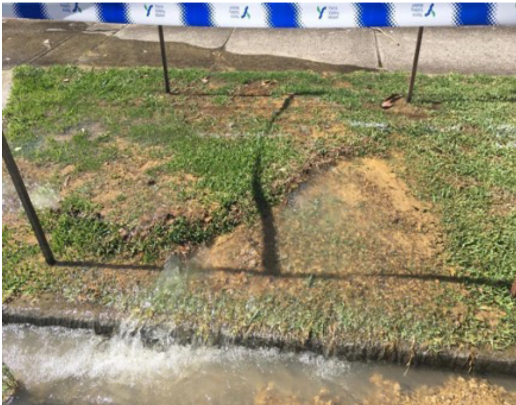
Figure 5.32. Stormwater pipe breakage in Donaldson Creek. Photographs by Ana C. Lara Heyns (2021)
