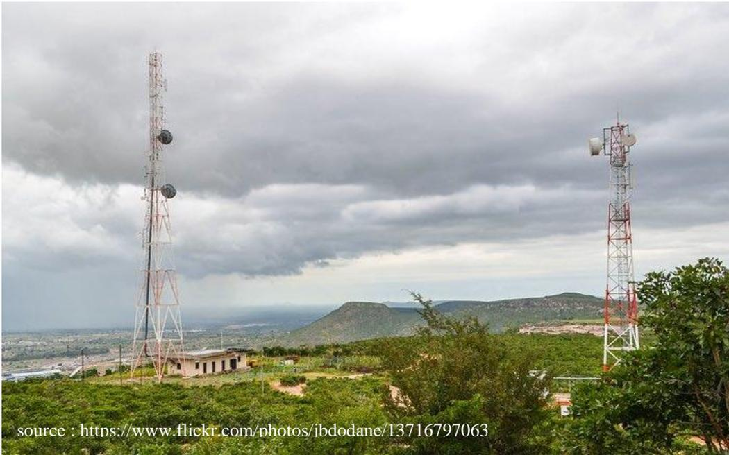
**Figure 1-1: Example of a commercial microwave link antenna tower, used in telecommunication networks.**
