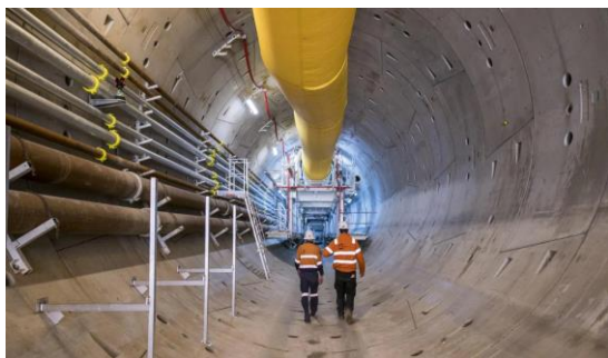
(c) Constructed tunnel by TBM
