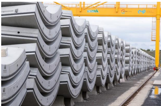
(a) Tunnel lining segments
