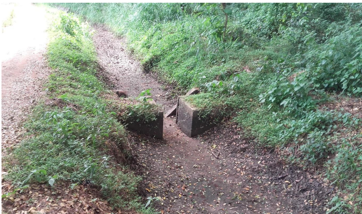
Figure 6.9. This concrete structure that regulates water distribution in field canals had been destroyed by farmers in an attempt to obtain extra water for their field. Photograph taken on site by the author with relevant permissions obtained.
