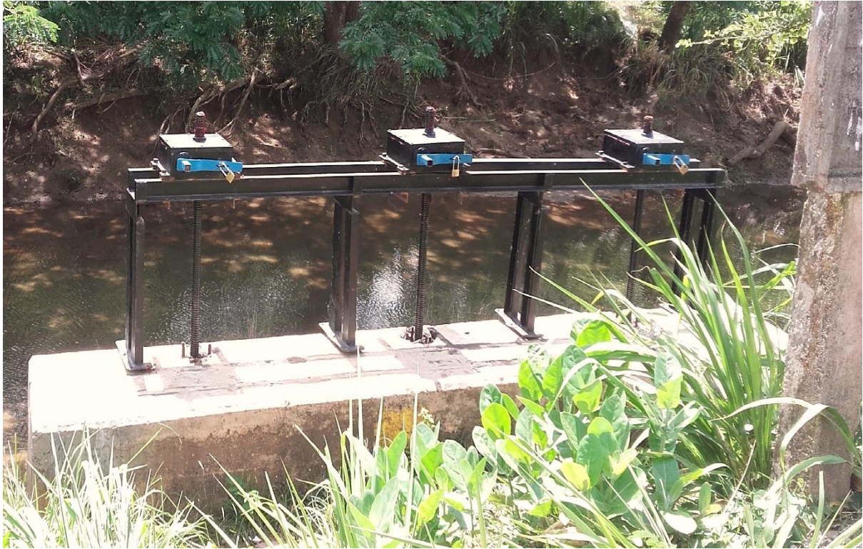
Figure 6.8. Turnout gates which regulate the diversion of water into individual farms. Farmers often break these locks to obtain more water for their fields. Photograph taken on site by the author with relevant permissions obtained.
