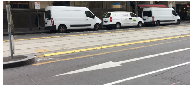
f. ROW C.3 tram lane separated by mountable kerb
