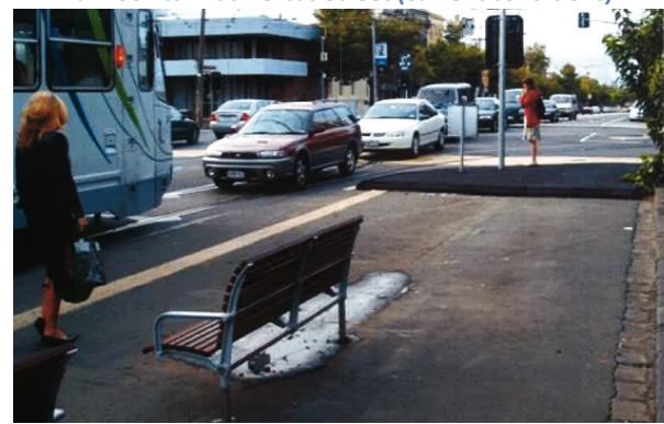
d. Far side kerb extension tram stop (during trial)
