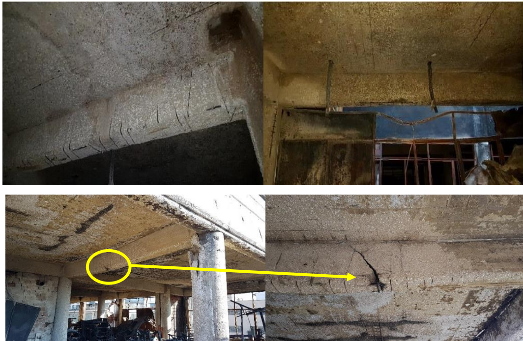
Figure 2.19: Spalling and visible reinforcement (Mehmet et al. 2018)
