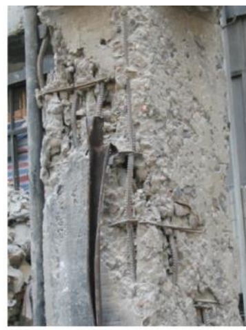
Figure 2.17: Spalling and visible reinforcement (Yi et al. 2015)
