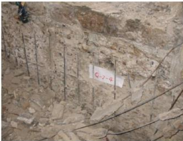
Figure 2.17: Spalling and visible reinforcement (Yi et al. 2015)
