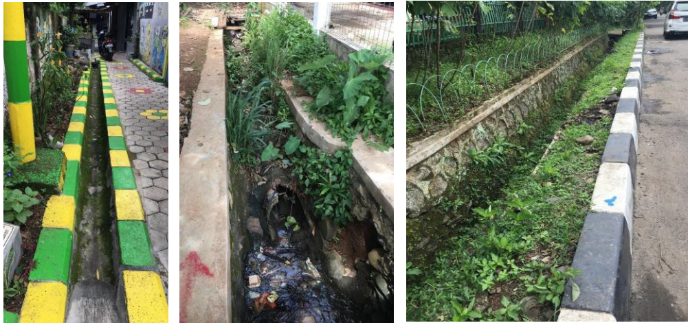
Figure 2- 9 Open drainage channels throughout Bogor, many adapted from the former irrigation system
