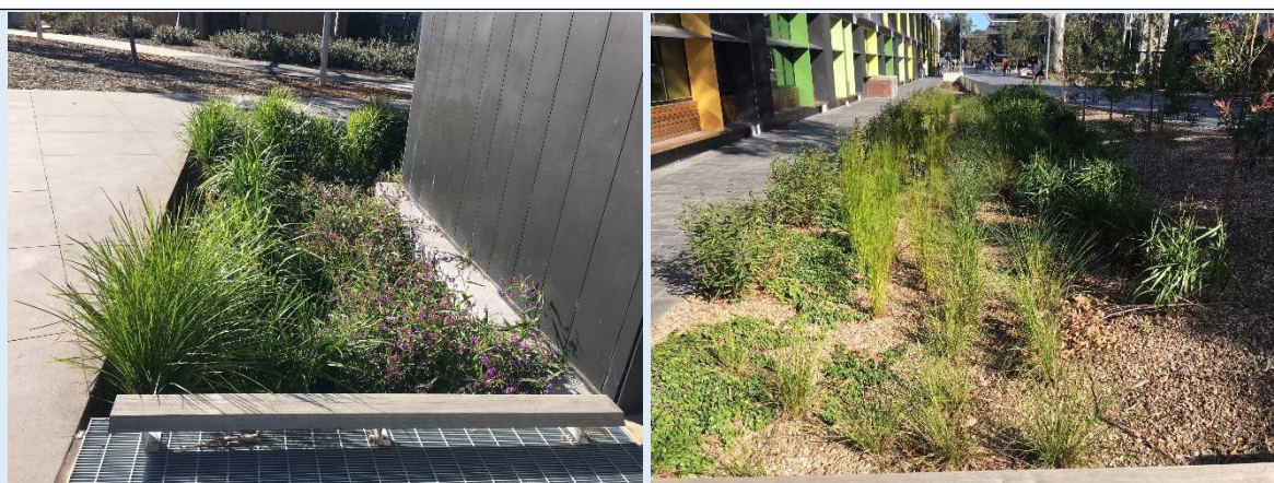
Examples of designs that allow water to runoff paved surfaces into sunken gardens passively; a simple raingarden design; at Monash University, Australia
