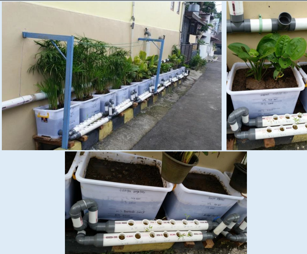
Demonstration biofiltration system treating greywater in Griya Katulampa
