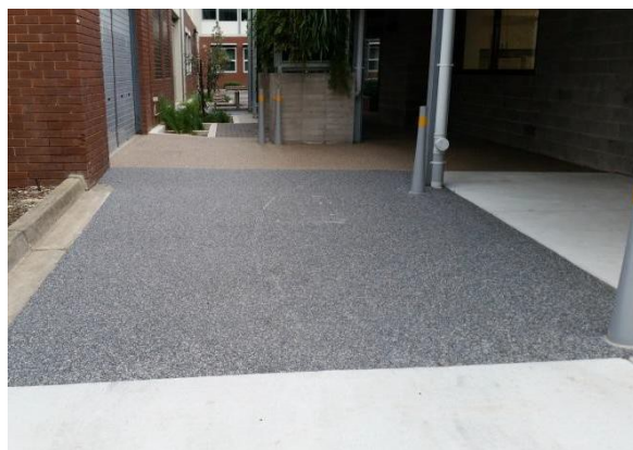
Figure 6- 17 An example of porous pavement at the entrance of a building at Monash University, Australia
