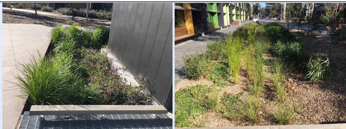
Examples of designs that allow water to runoff paved surfaces into sunken gardens passively; a simple raingarden design; at Monash University, Australia
