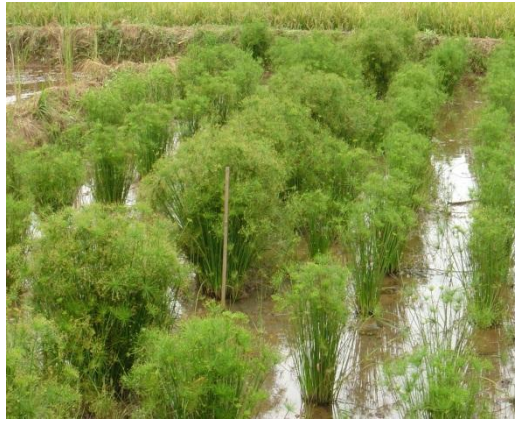
Figure 6- 10 A surface flow wetland in Indonesia; Image: Dr. Cynthia Henny and research team, LIPI Limnology
