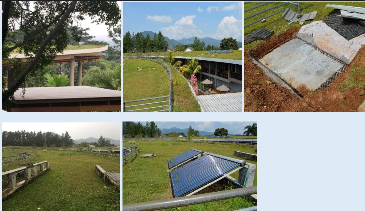
Green roof system covering the Hotel Neo Savana in Sentul City. Image at top right shows an access panel opened to illustrate the depth of substrate and layers beneath; concrete, waterproofing, geomesh, geopolymer, soil and grass. Solar panels are also located on the roof (shown in centre bottom image) Source: Images provided by Raul Marino
