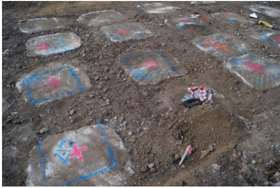
Figure 3.12. Column heads following removal of the hardstand (17 April 2013)
