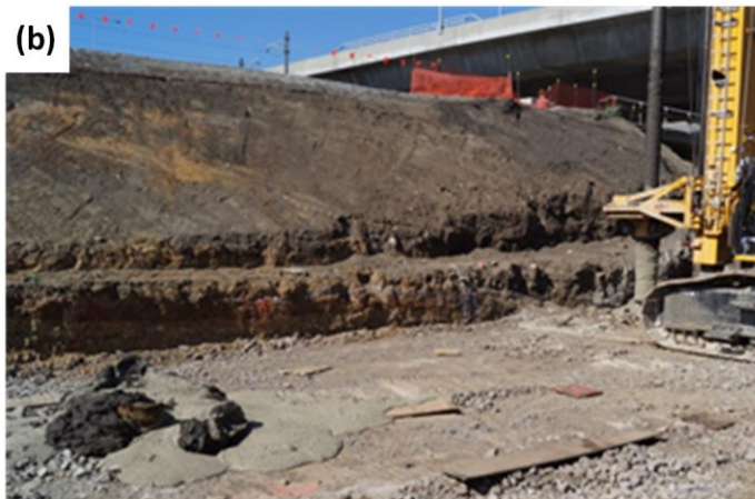
15 March 2013 – Stage 1 ground improvement works, temporary batter slope and exposed Historic Embankment Fill in vertical cuts (approximate R.L. 2.0 to 2.7 m)
