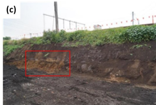
29 June 2013 – embankment construction, exposure of existing rail embankment (R.L. 4.3 m). Fill material is inferred to be derived from weathered Tertiary aged Older Volcanics Basalt.
