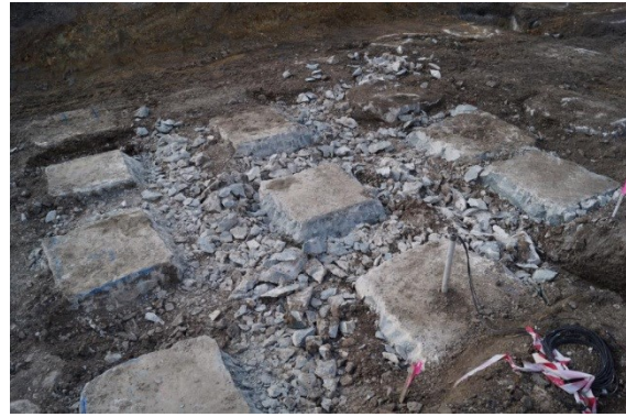
Figure 3.13. Area #2 column heads after “breaking-back” (19 April 2013)
