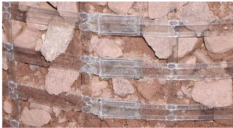
Figure 2.16: Conventional welding of horizontal geogrid ribs
