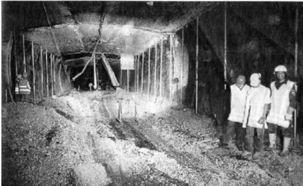
Figure 1.2 The Tauern Tunnel fire in 1999. Adapted from (Leitner 2001)
