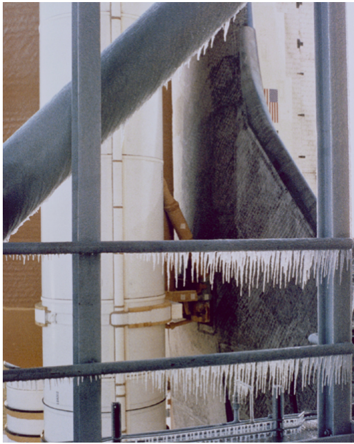
(a) Ice on the Challenger launch gantry. ©NASA, http://grin.hq.nasa.gov/ABSTRACTS/GPN-2000-001348.html
