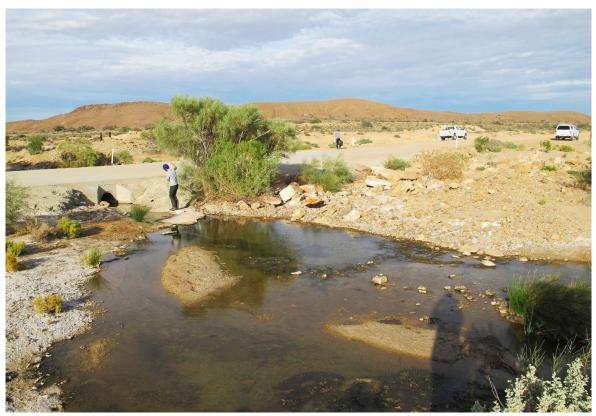
**Figure 12**. A pool formed as a result of a raised roadway in the Lake Eyre Basin, in which several fish species were found. While a culvert is present, it was disconnected from the main pool.
