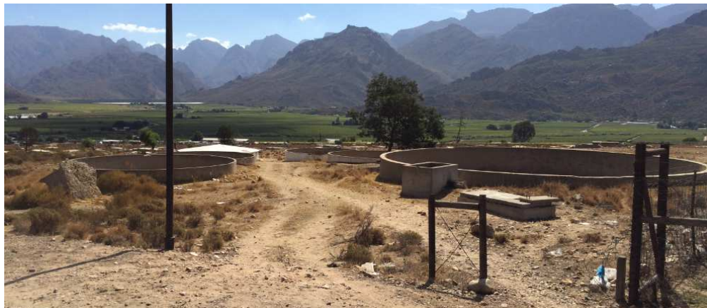
Picture 6: Drinking water reservoirs for Orchards - One out of five was functional (covered with a corrugated iron)
