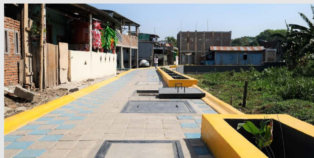
Water and sanitation intervention for a neighbourhood in Makassar comprising below-ground tanks for temporary storage, and septic tanks and constructed wetlands for sewage treatment. The intervention also included a raised pathway and drainage.
